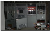
The bottling company installed 24-inch large-format IR windows in main breaker huss cabinets
